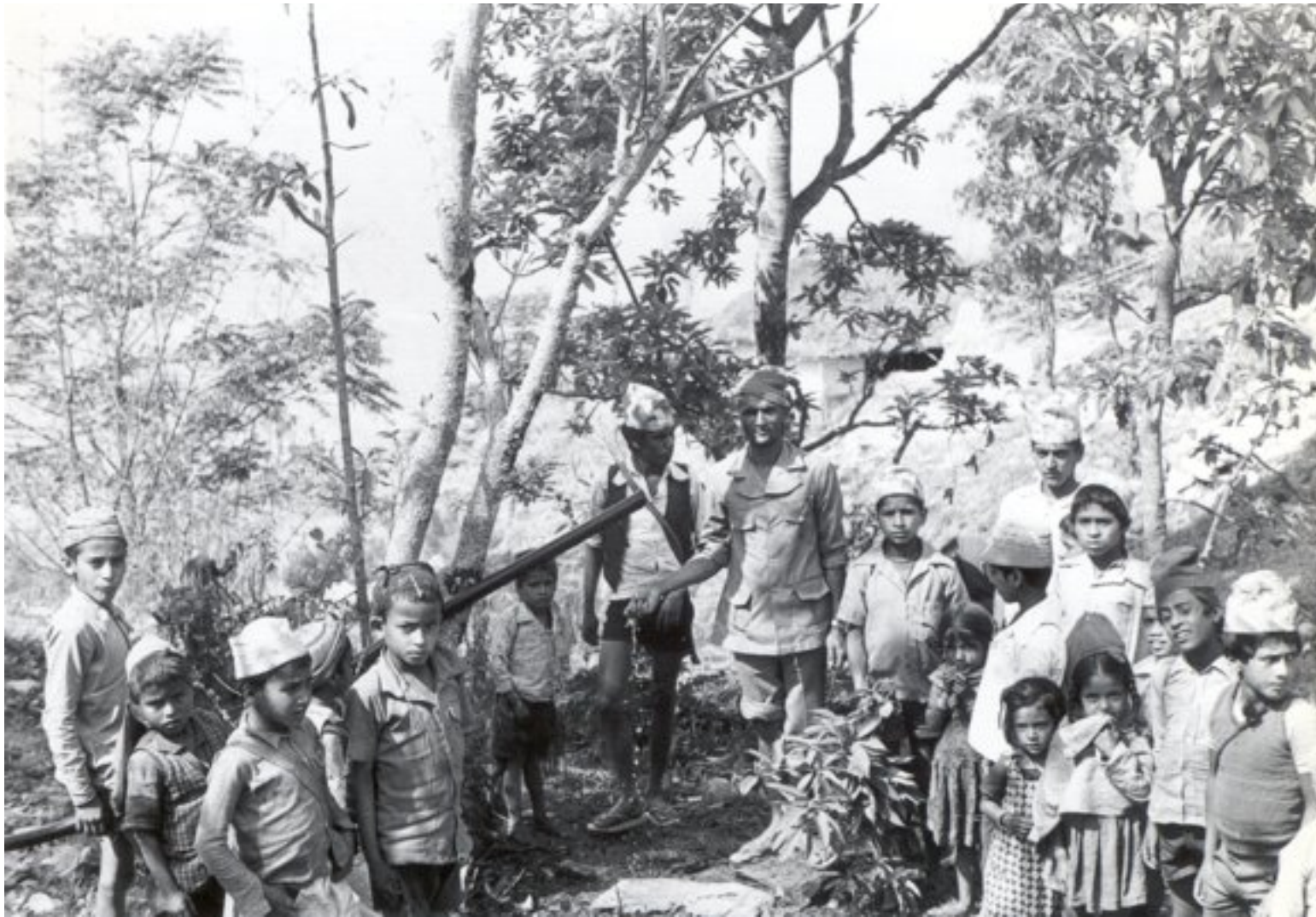
The pipeline was buried along this area. Some of the pipe can be seen at the left. Netra Narayan Subedi, the teacher, can be seen standing in the middle.
