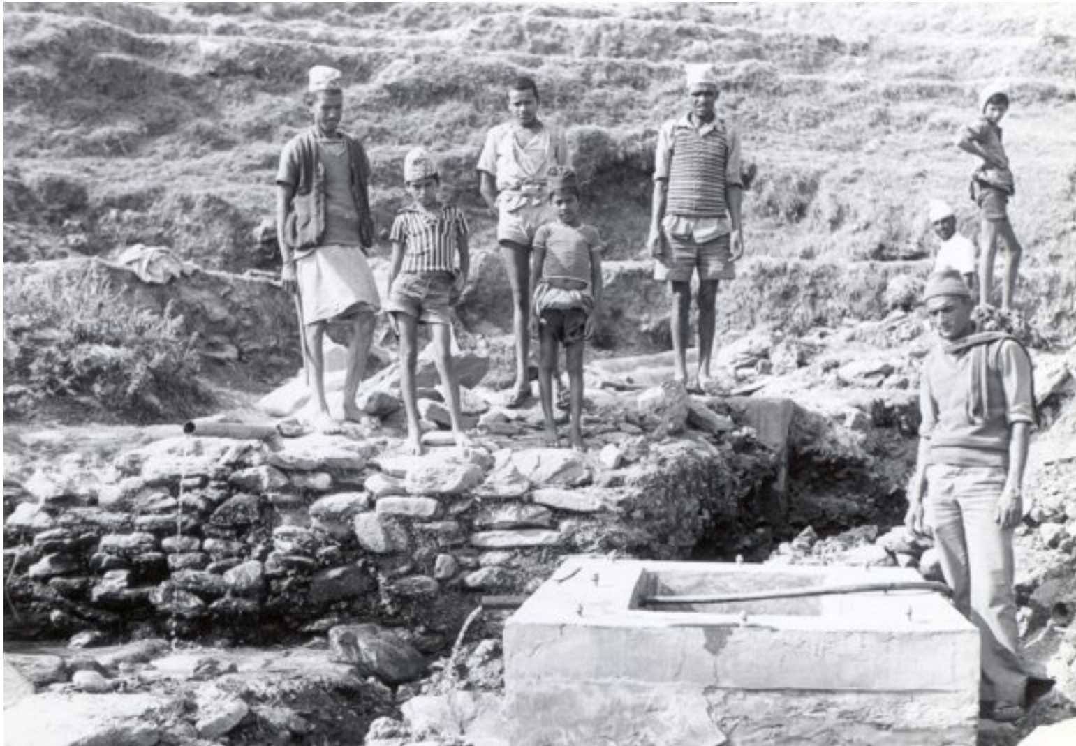
The new tank is shown, as yet uncovered, by the inlet gallery. The other two tanks were fed in series from this source tank.
