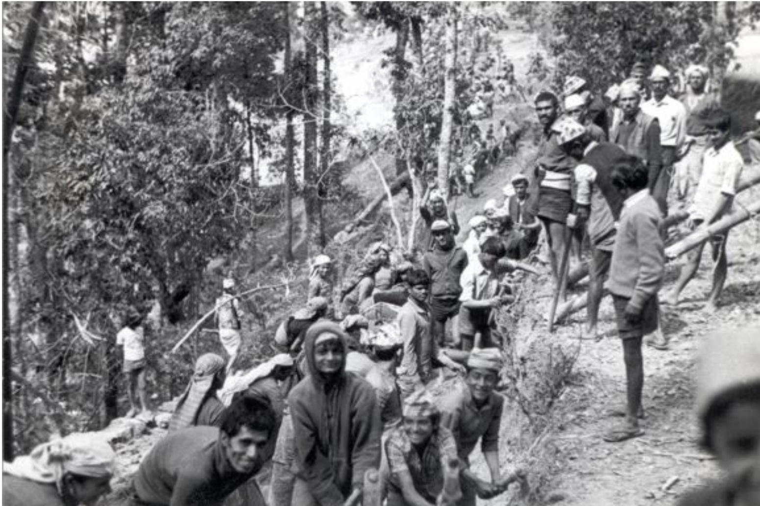
Villagers working on a new motor road (never finished at this location). Nearly all work is by manual labor.
