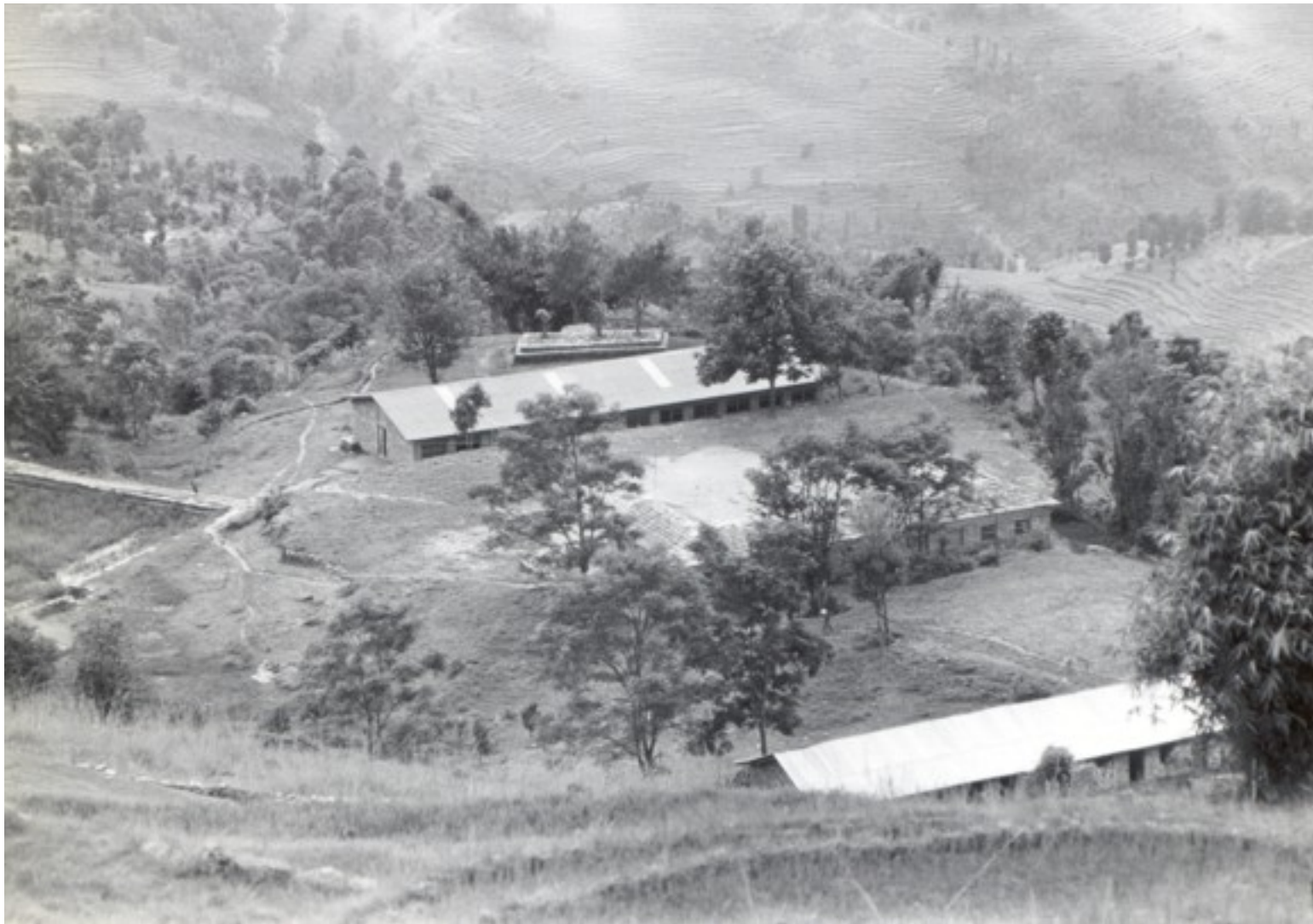
This is another photo of JS Secondary School campus looking from near Devisthaan. The area stripped of grass in the center is where students normally play volleyball. Note the chautara in the background.
